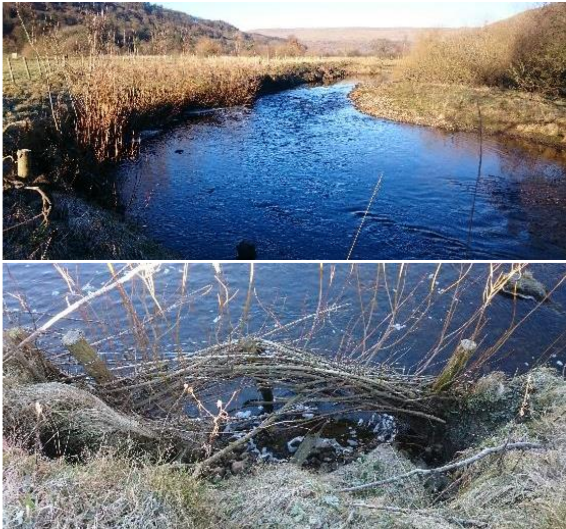
Fig 3. A short section of willow spiling to reduce erosion scour on the RB (upper). While this has started to grow and the roots will help retain the structure, the tail end of the spiling has been undermined by flow and scour is beginning again (lower). The hole should be packed with living willow brash and wired into position, continuing the brash ~2m further d/s to prevent re-occurrence. Living willow whips inserted through the spiling at the waterline and from the river side will help soften the force of the water working against the spiling. The roughness and diffuse nature of brash often makes it more applicable than willow spiling for bank protection work on upland rivers.
