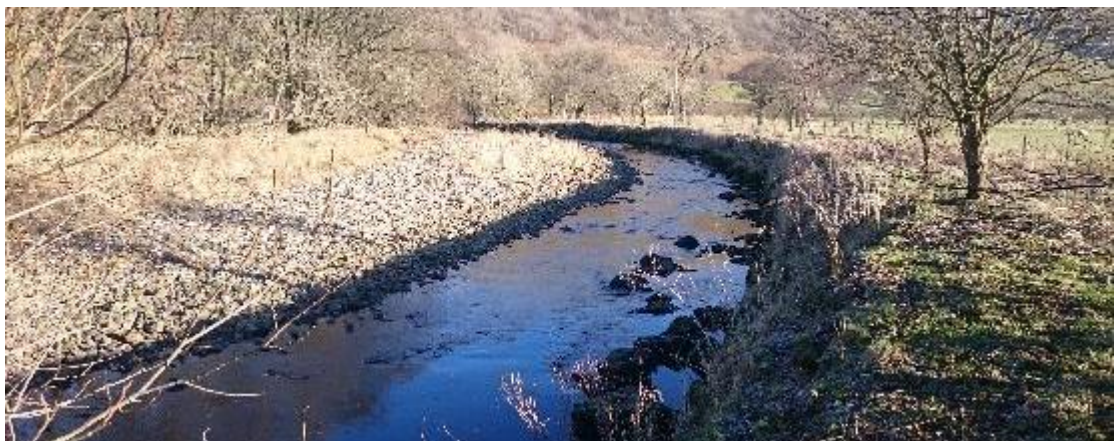
Fig 14. Long, sweeping bend resulting from channel realignment and rock armouring of the RB; devoid of cover, the RB would benefit from tree planting. These unnaturally long, sweeping bends tend to create elongated riffles and prevent pool formation.
