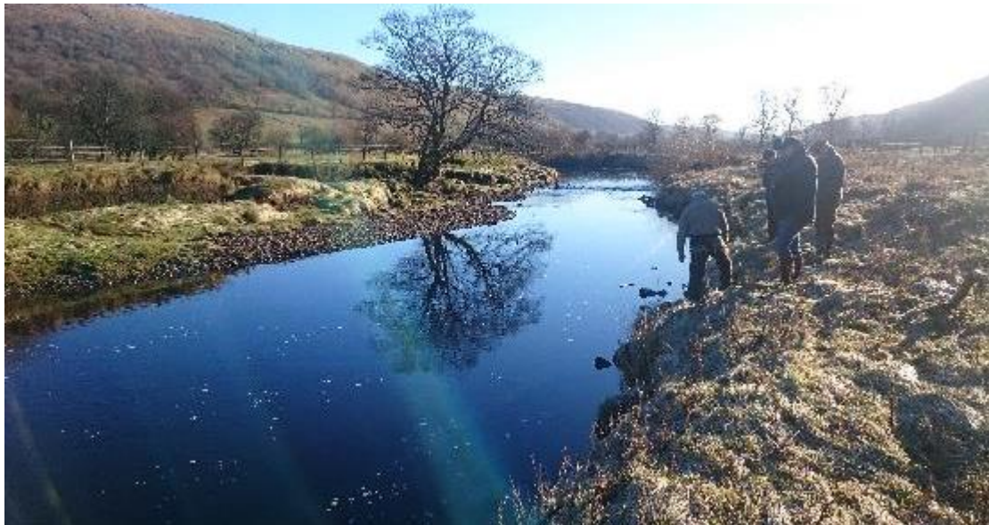
Fig 5. The d/s end of a very long straightened section (about mid-way along the lower Buckden length) where armouring on both banks is obvious. The armouring and associated drystone wall have failed in several locations and introduced large boulders which bounce the water flow away from the edge, actually introducing some sinuosity at low flows. This could be encouraged in further locations. The banks require some willow whip planting as there is a distinct lack of cover. NB: mink tracks were observed here.
